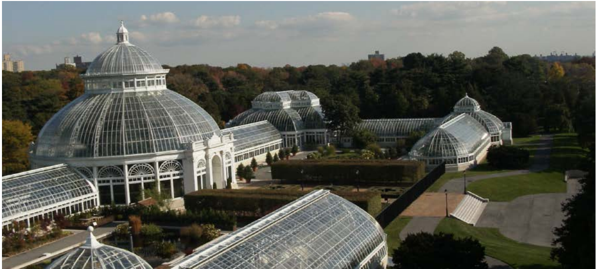
The Dome's compression ring needs replacement.
