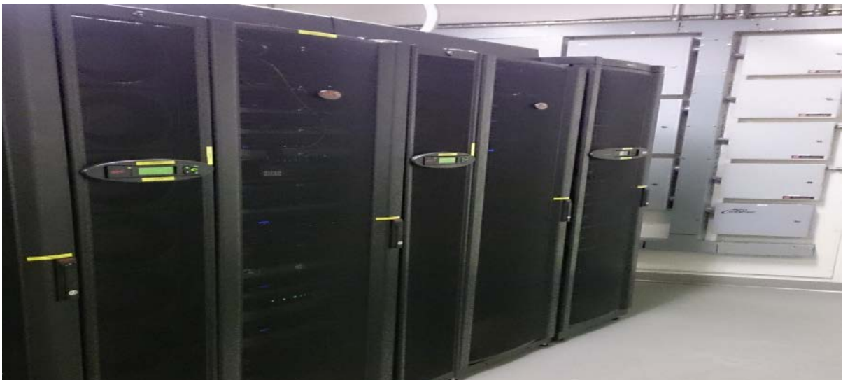
Networking and data storage equipment
