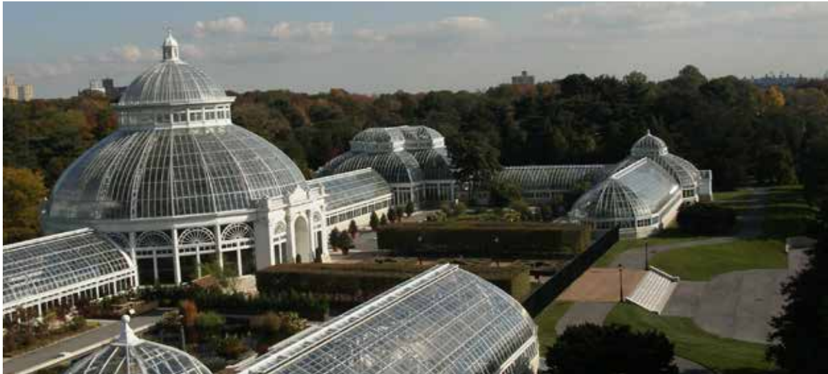
The Dome's compression ring needs replacement.
