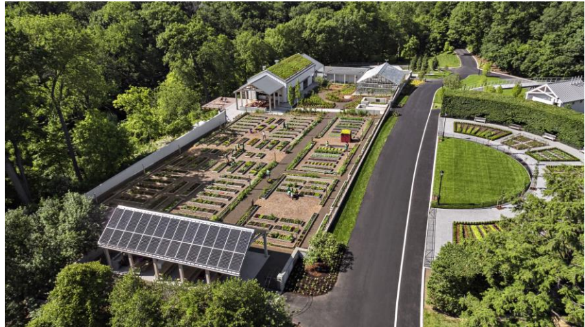
The indoor-outdoor campus of the new Edible Academy now allows NYBG’s edible gardening program to operate year-round. © Robert Benson Photography
